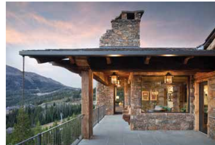
The dining terrace, built with radiant Pennsylvania bluestone, features a custom railing with an aspen leaf motif. A crane was used to place the grand, rustic chimney.
